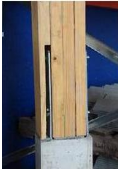
After installation of trim board
