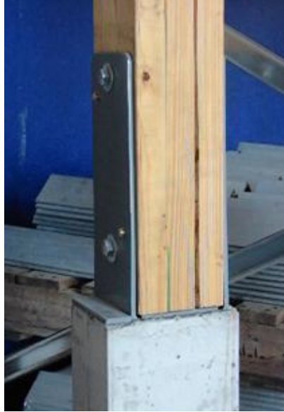
Before installation of trim board
