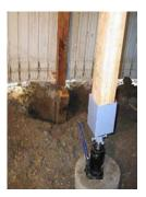
**6.** Clean out post hole to provide a level, compacted base for the pre-cast concrete pad. Sakrete or ready mix concrete can also be used for post base.
