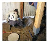
**7.** Install pad and measure the Perma-Column for exact clearance needed. **Note:** Perma-Column length may vary.
