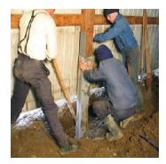
10. Install 1/4" x 3" wood lags. Drill and install (2) 1/2" bolts.
